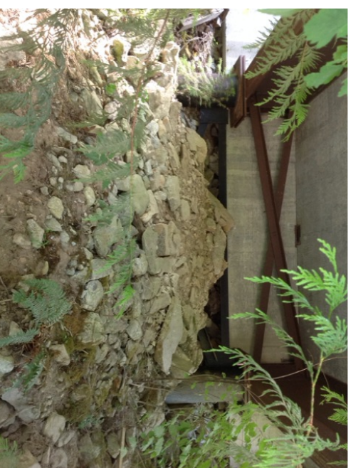
Right Bank Abutment when facing downstream
